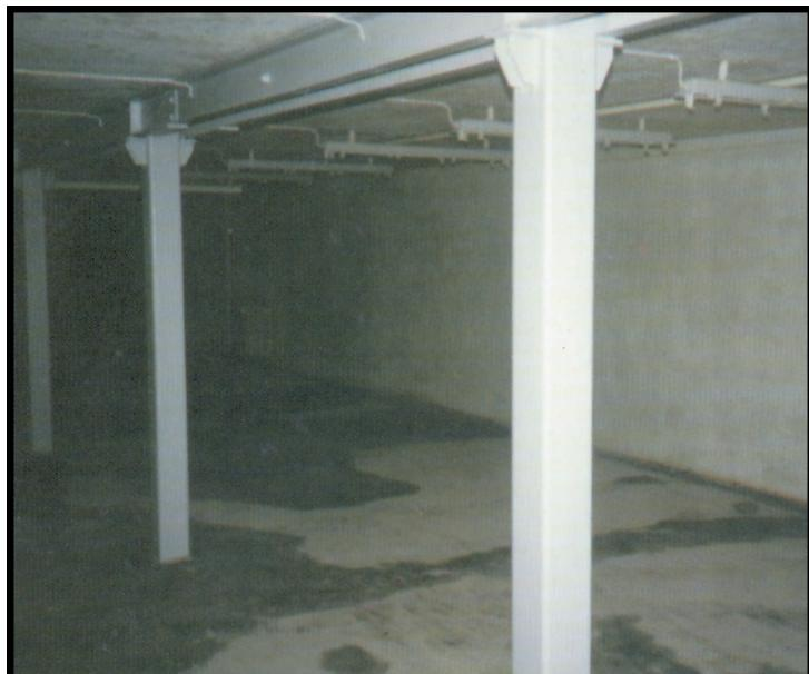
All steelwork was thoroughly cleaned by manual means and then primed with Unitech M.C. Primer followed by one single application of Pyro-Tech S.P. by spray.
